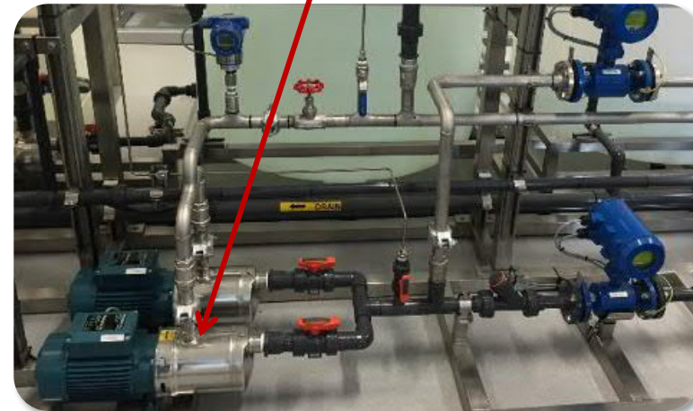
Pump in the plant
